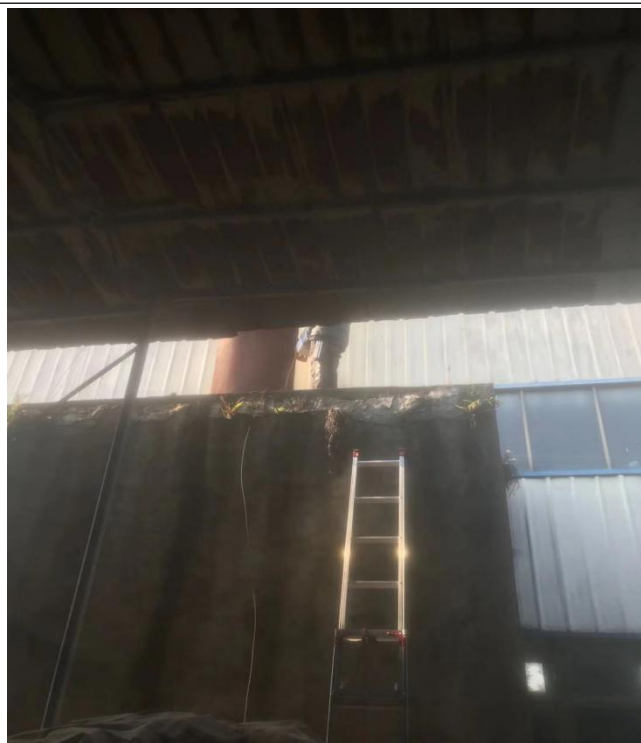
喷涂废气出口1#
